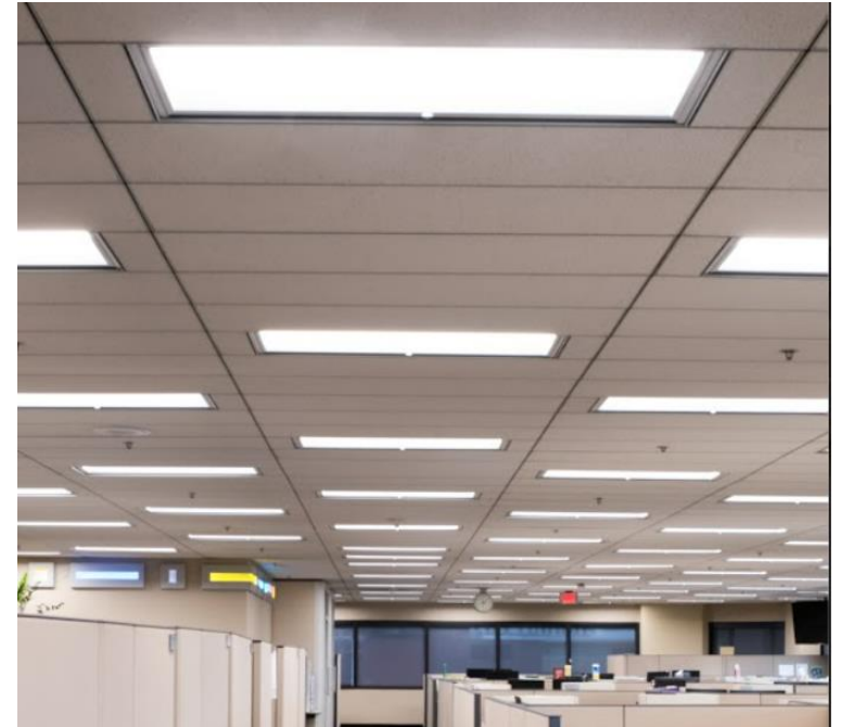
Troffer door kits with integrated Bluetooth mesh enabled sensor controller
